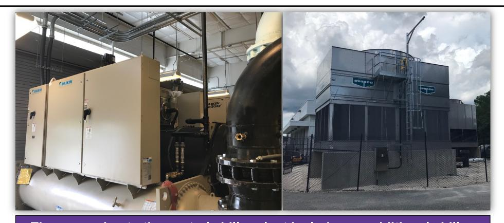
The expansion to the central chiller plant includes an additional chiller, and cooling tower in order to maintain compliance with the University's Campus Master Plan Policy to provide redundant cooling across campus. With the addition of the Applied Research Center, redundant cooling was taxed, so the additional chiller brings the University back to a state of n + 1 redundancy.
