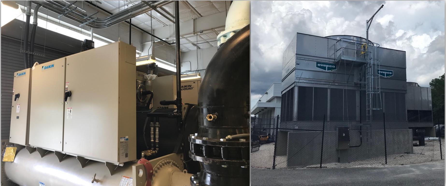
The expansion to the central chiller plant includes an additional chiller, and cooling tower in order to maintain compliance with the University's Campus Master Plan Policy to provide redundant cooling across campus. With the addition of the Applied Research Center, redundant cooling was taxed, so the additional chiller brings the University back to a state of  $n + 1$  redundancy.
